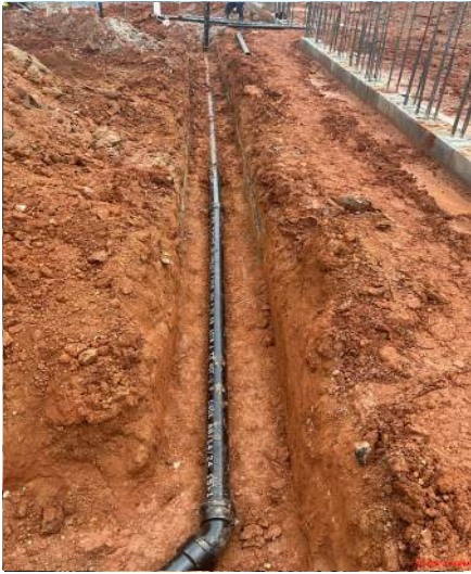
Sanitary sewer installed under slab
