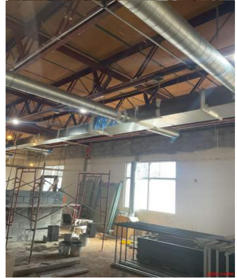
Ductwork completed in cafeteria
