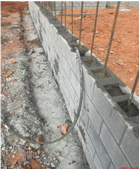
Grouting 8" block around stage walls
